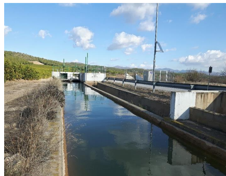
Figure 2.3 - An example of an irrigation canal where water requires pumping to the fields (Liria, Spain)
