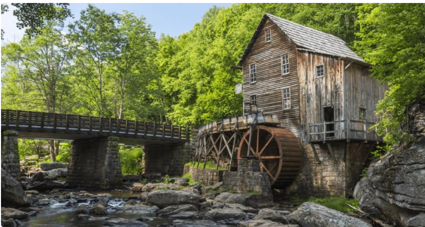
Figure 5.1 – Example of a traditional stream waterwheel installation [14]
